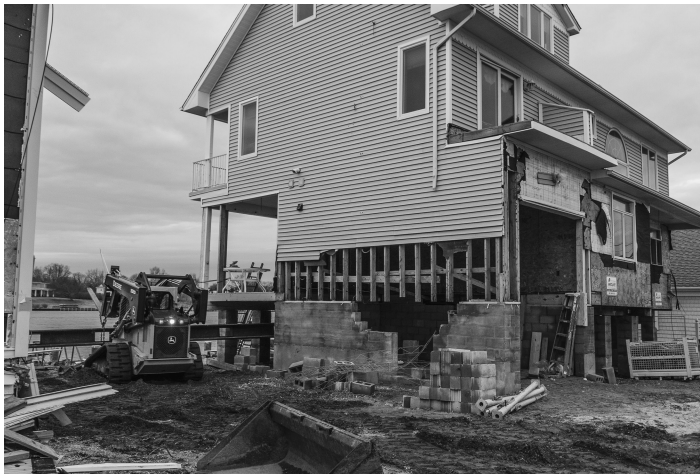
FIGURE 2.6 Sea Bright, New Jersey: Construction crews are elevating this house damaged during Hurricane Sandy. Elevation, or raising the base floor above expected flood heights, is one way to mitigate flooding for a home situated in a flood zone.
