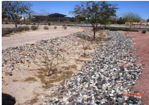
Sediment Deposit at Points of Flow Interception
