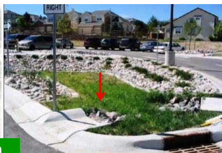
Construction of LID Rain Garden
