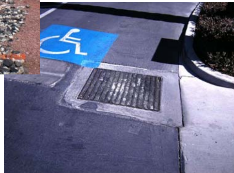
Sediment Deposit at Points of Flow Interception
