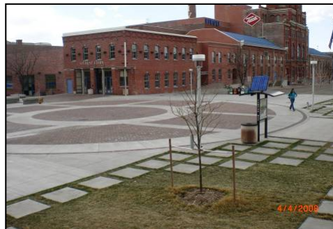
Porous Pavements in UC-Denver Campus
